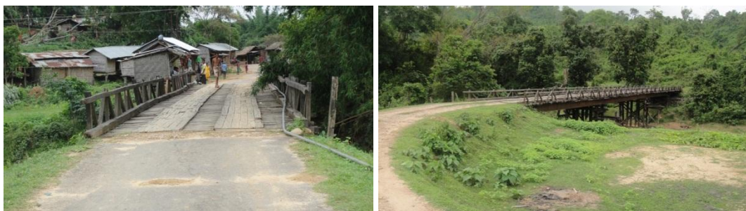
Two of the many Semi Permanent Timber Bridges (SPT) in the State. These are vulnerable to flash floods & require regular repair and decking replacement. Many of these have been replaced by RCC bridges in the 11 th Plan, many more remain
