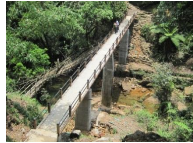
RCC footbridge built to connect a border village
